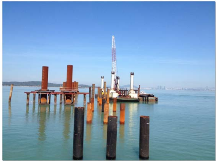
P51~P52構台鋼管樁施工
