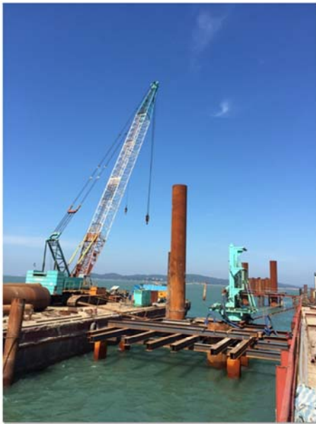
P52外套鋼管施工
